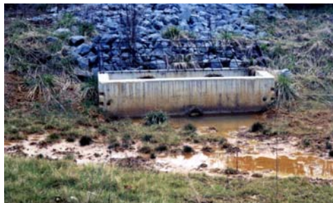
Brown water should NEVER leave a pond or a basin like this one above. If you see a pond overflowing with brown water or leaking brown water, take a picture! If a pond is holding brown water, that is ok ( see below ).
