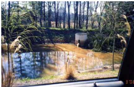
Brown water should NEVER leave a pond or a basin like this one above. If you see a pond overflowing with brown water or leaking brown water, take a picture! If a pond is holding brown water, that is ok ( see below ).
