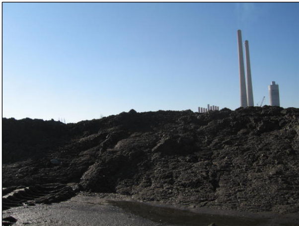
Kingston Fossil Plant – Coal ash contains selenium and it was dumped into our waters when the spill occurred.
