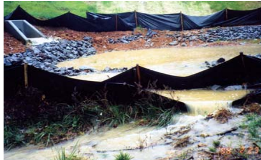
These black structures are called silt fencing. No water, mud or dirt should ever leave a silt fence. If you see water, mud or dirt on the other side of a silt fence. Take a picture!
